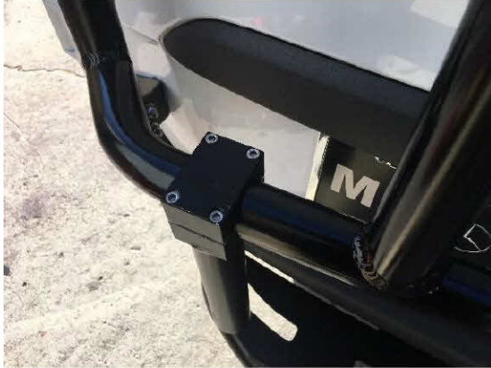
Figure 1: Bolt-On Supports Loosely Bolted to Lower Crossmember
