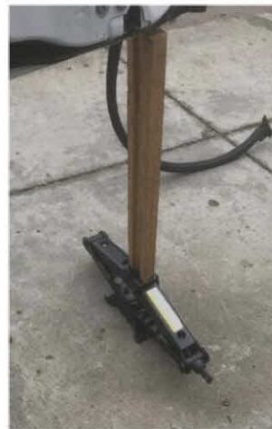
Figure 2: Support Door Prior to Installation
