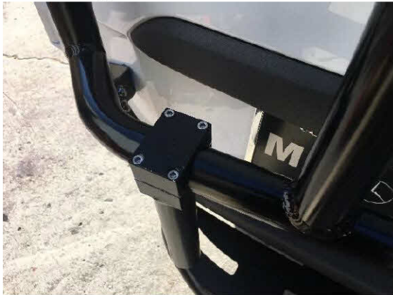
Figure 1: Bolt-On Supports Loosely Bolted to Lower Crossmember
