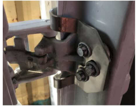
Figure 5: Inside View of Installed Upper Hinge
