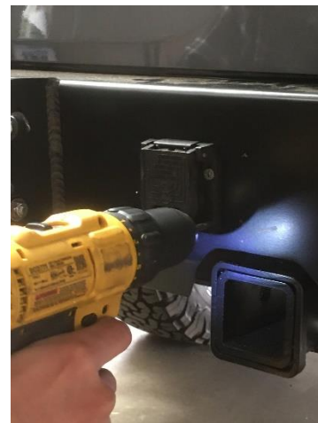
Figure 15: Installation of the trailer plug
