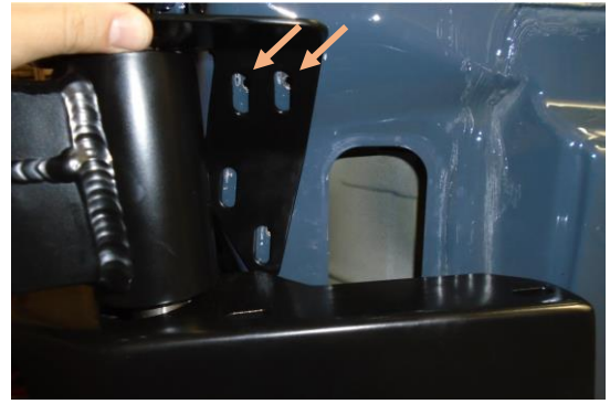
Figure 11: Drilling for Axle Support Bracket
