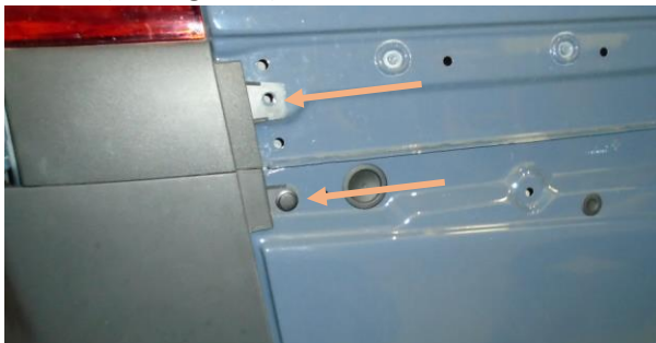
Figure 6: Plastic Rivets Underneath the Side Panel
