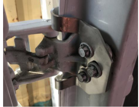
Figure 5: Inside View of Installed Upper Hinge
