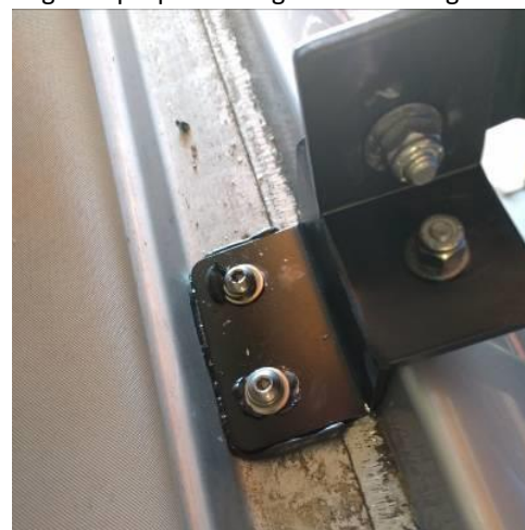
Figure 2: Upper Attachment Assembly Installed into the Roof Gutter
