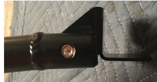
Figure 2: Ladder Attachment to Upper Brackets
