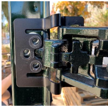
Figure 3: Bracket Installed Over Factory Hinge
