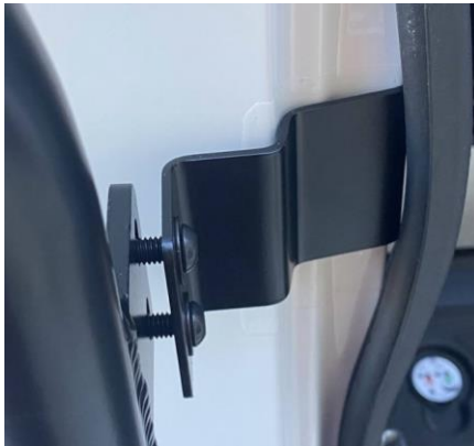
Figure 16: Example of gap between bracket and product
