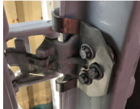
Figure 5: Inside View of Installed Upper Hinge
