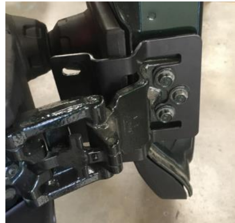
Figure 6: Inside View of Installed Lower Hinge Bracket
