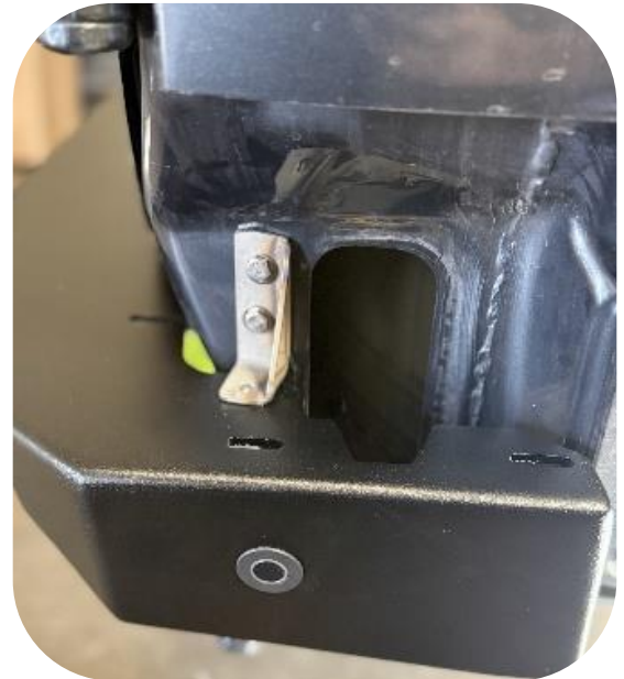
Figure 12: Support Bracket Installed
