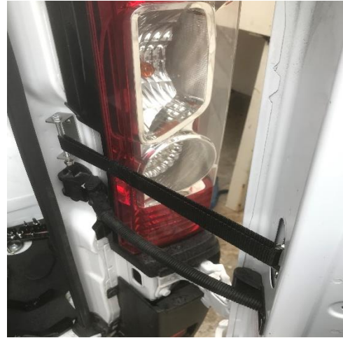
Figure 17: Completed Door Strap Installation
