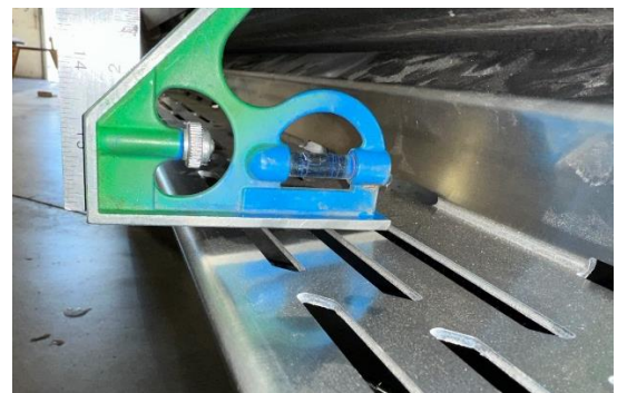
Figure 3: Verification that the Step is Level
