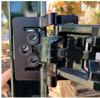
Figure 3: Bracket Installed Over Factory Hinge
