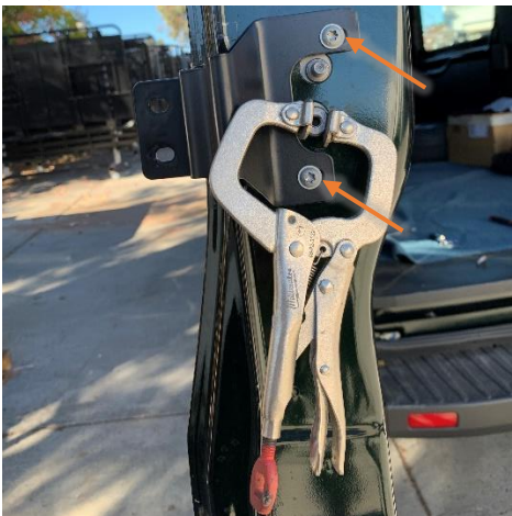
Figure 8: Inner Driver Door Bracket Installed
