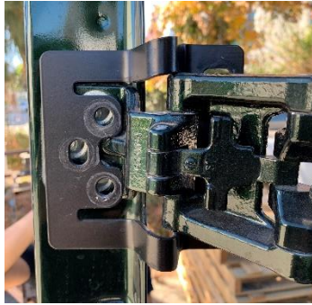
Figure 3: Bracket Installed Over Factory Hinge
