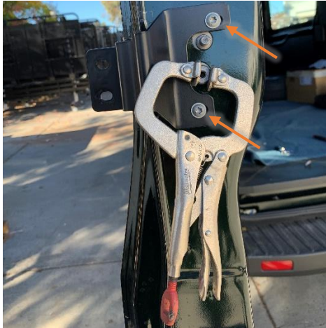
Figure 8: Inner Driver Door Bracket Installed
