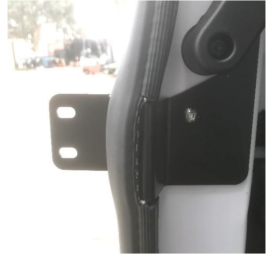
Figure 15: Installed Weather Stripping After Modification
