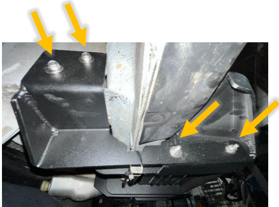
Figure 19: Installation of Front Passenger Mounting Bracket
