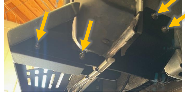
Figure 10: Installation of Front Passenger Mounting Bracket
