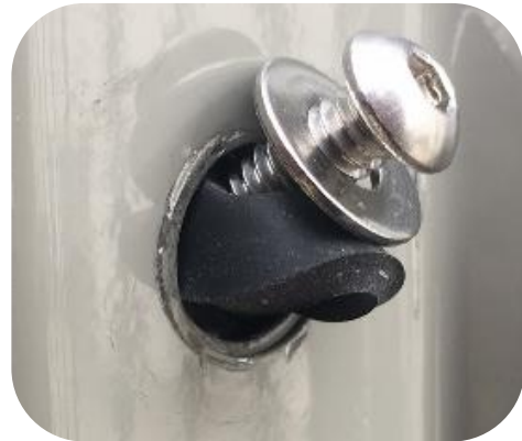
Figure 13: Installing the Cushioned Washer
