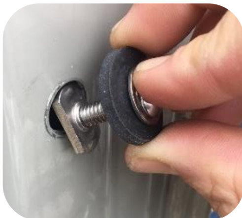
Figure 12: Installing the Nut
