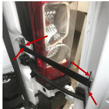
Figure 18: Completed Door Strap Installation
