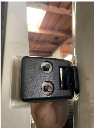
Figure 25: Upper Hinge Bolt Routing
