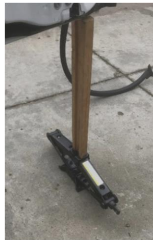
Figure 2: Support Door Prior to Installation
