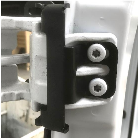
Figure 7: Inside View of Installed Upper Hinge Bracket
