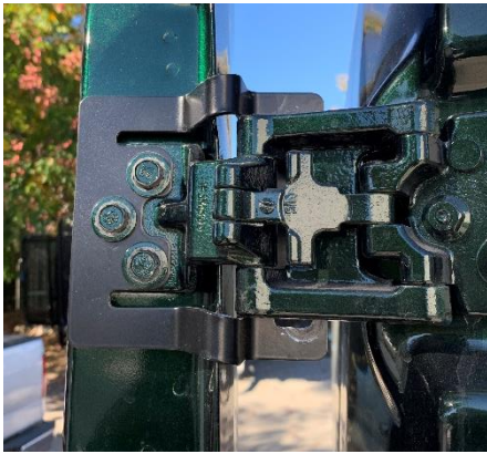
Figure 4: Inside View of Installed Upper Hinge Bracket
