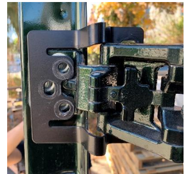
Figure 3: Bracket Installed Over Factory Hinge
