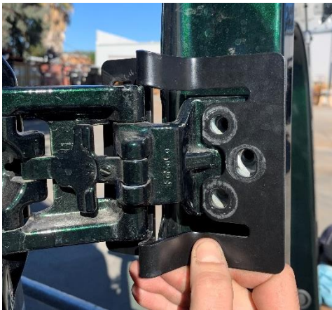
Figure 3: Bracket Installed Over Factory Hinge
