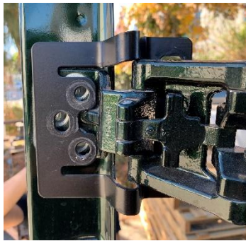
Figure 3: Bracket Installed Over Factory Hinge
