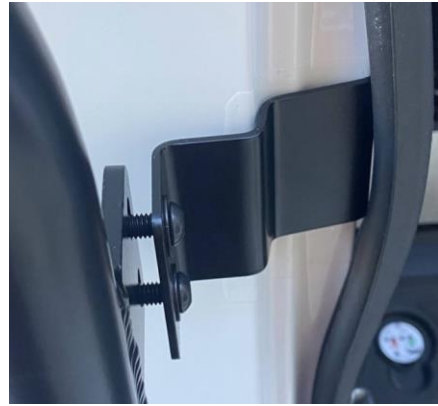
Figure 16: Example of gap between bracket and rack
