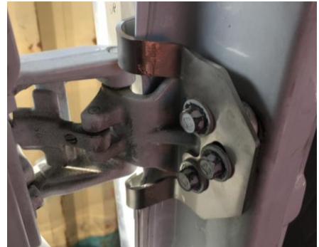
Figure 5: Inside View of Installed Upper Hinge
