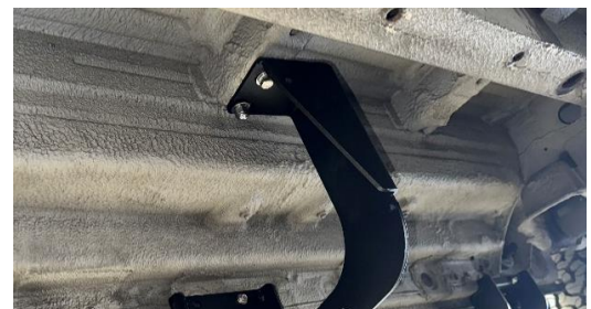
Figure 3: 'J' Bracket Installed onto Bolt Plate
