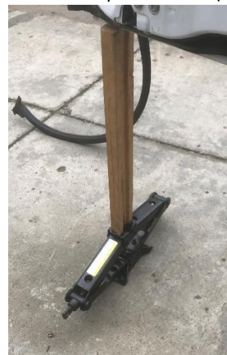
Figure 2: Support Door Prior to Installation
